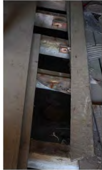
Whitewashing on underside of floor joists. Photo by Jennifer Glass.
