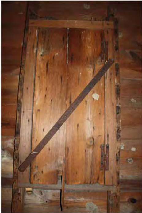
Exterior view of east window and shutter with H-hinges and iron bar. Photo by Jennifer Glass.
