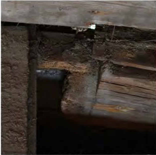
Interior view of sill cutout for chimney. Photo by Jennifer Glass.
