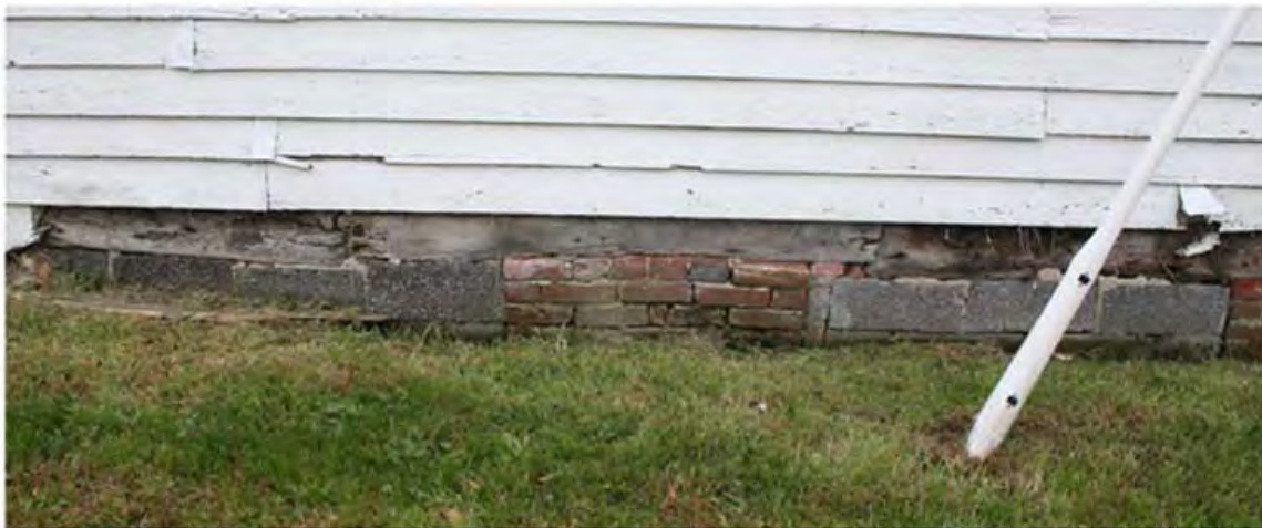
Brick pier foundation with concrete block infill. Photo by Jennifer Glass.
